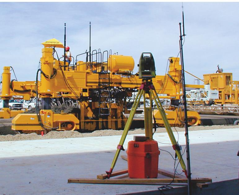
**A.S. Horner averaged about 1,200 cubic yards per day in full-production mode using a stringless 3D laser-control system developed by GOMACO and Leica when replacing hangar aprons at Kirtland Air Force Base.**
