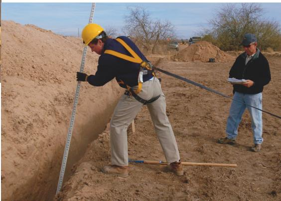
**Wearing a safety harness that's tethered to the lifting eye on the bucket of an excavator (with engine running), Andy Nicolas takes trench measurements as Gary Tindall records.**
